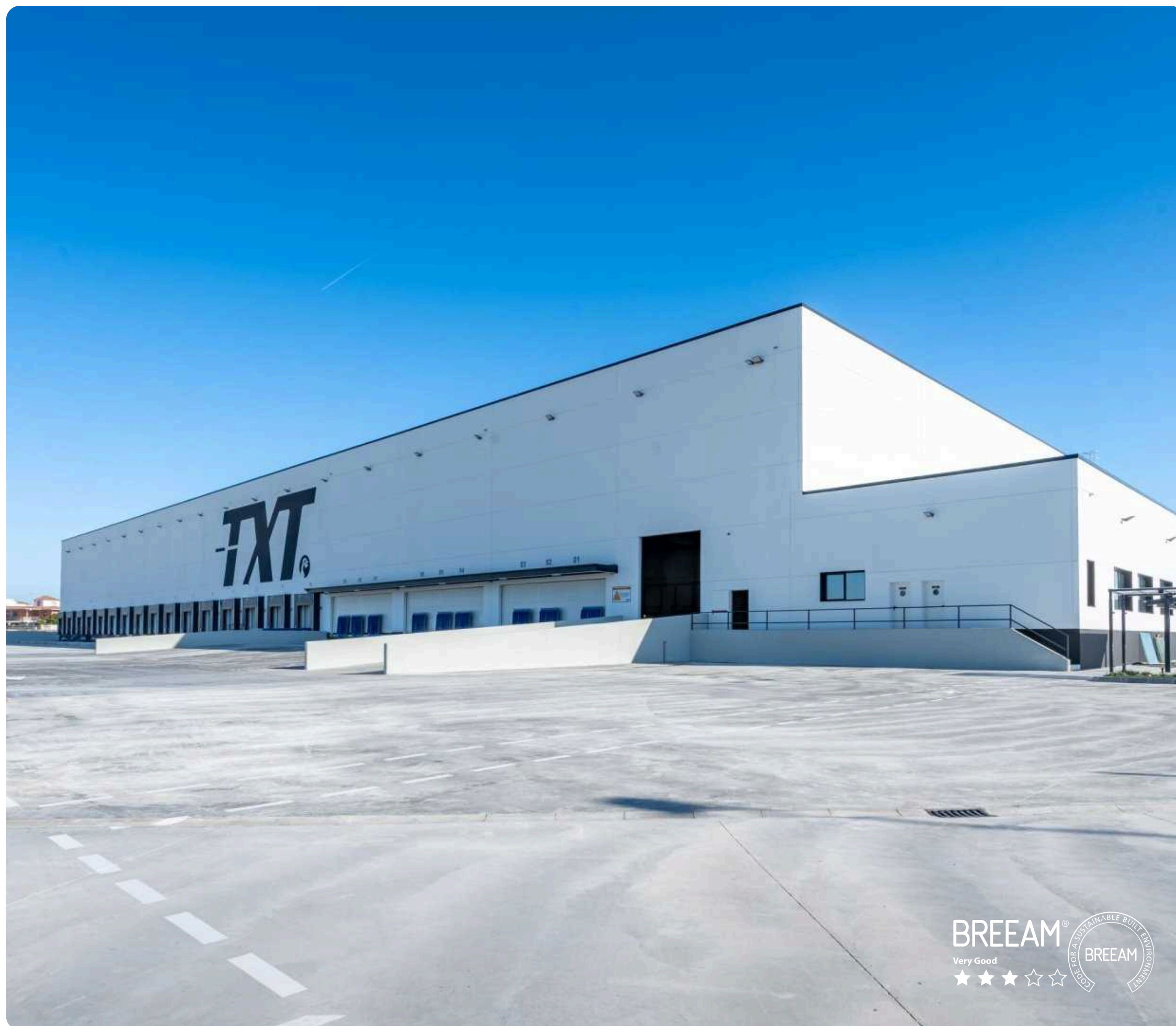
ACCOLADE FUNDS PARK SEVILLA
