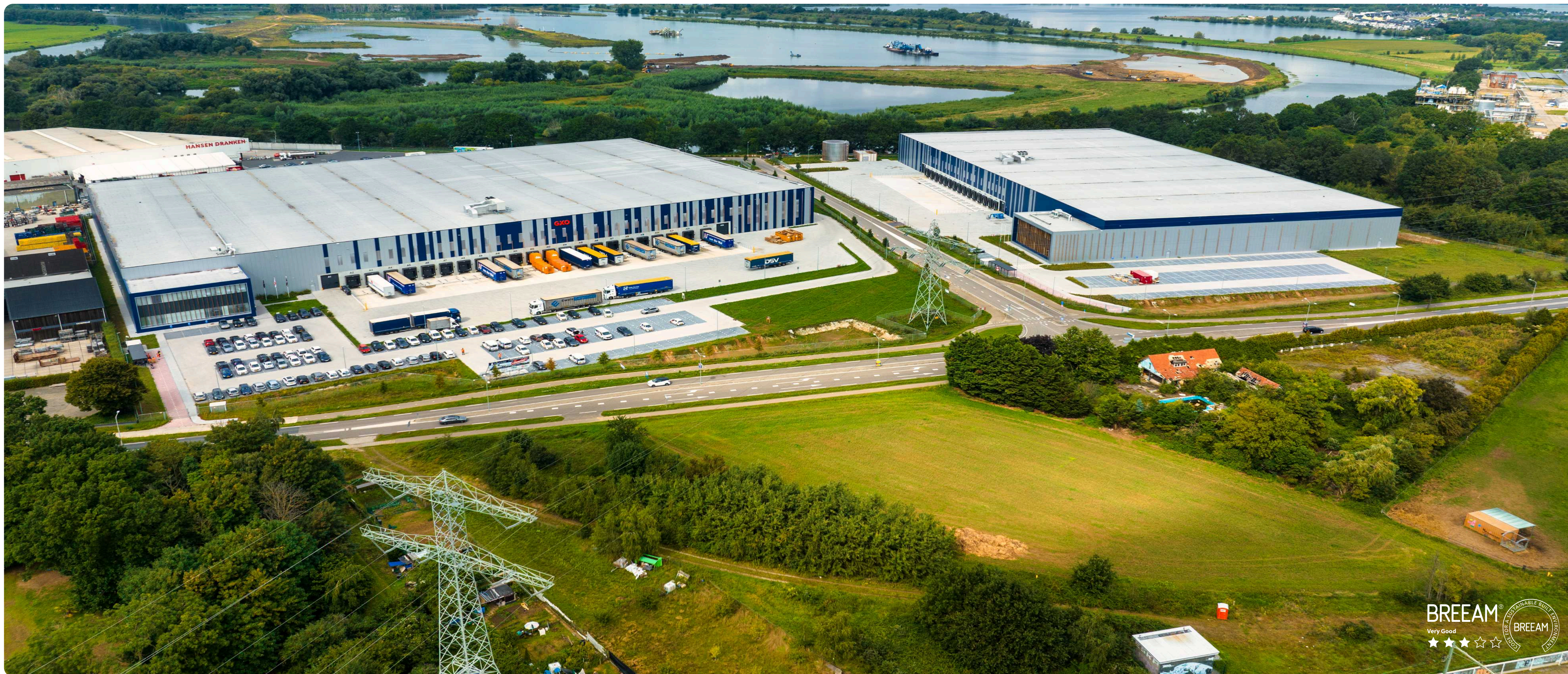
ACCOLADE FUNDS PARK ROERMOND
