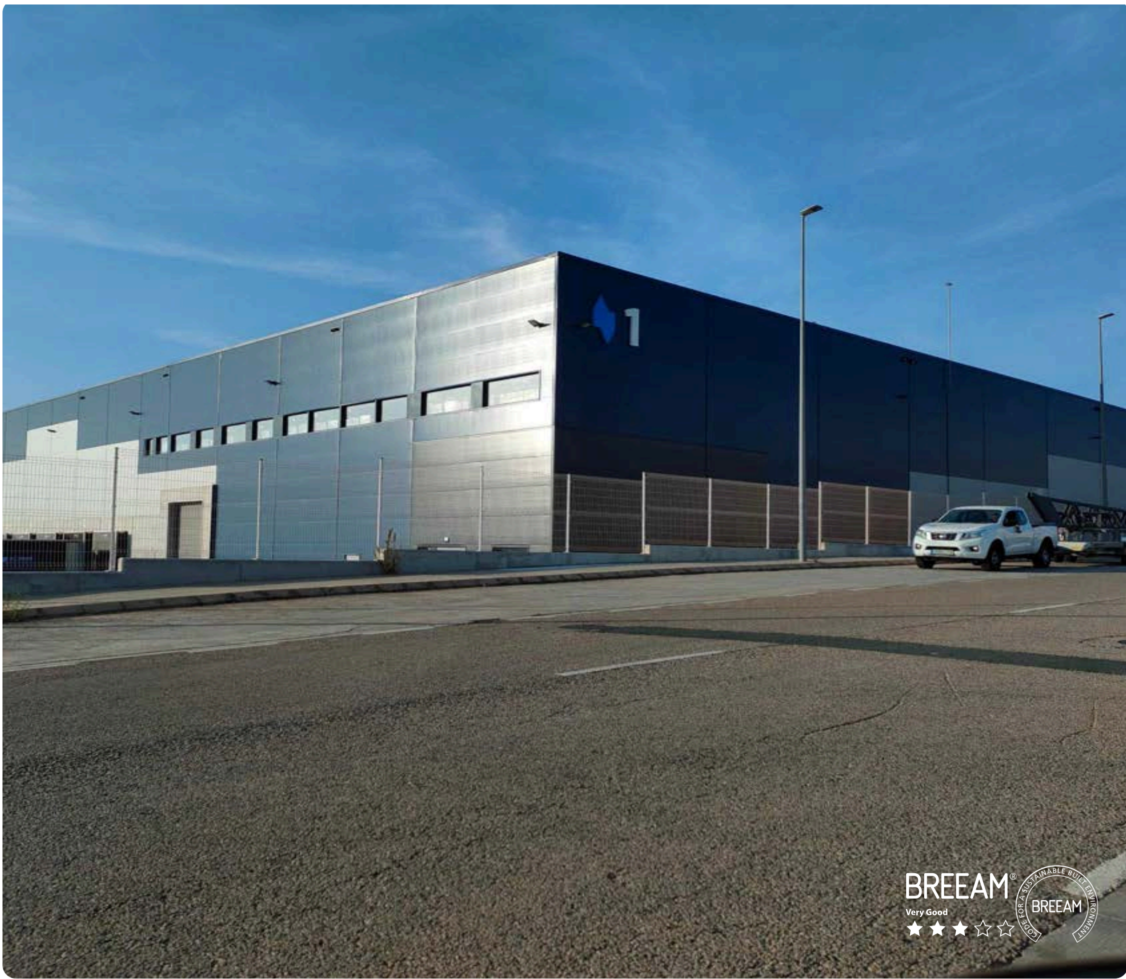
ACCOLADE FUNDS PARK VALENCIA PICASSENT
