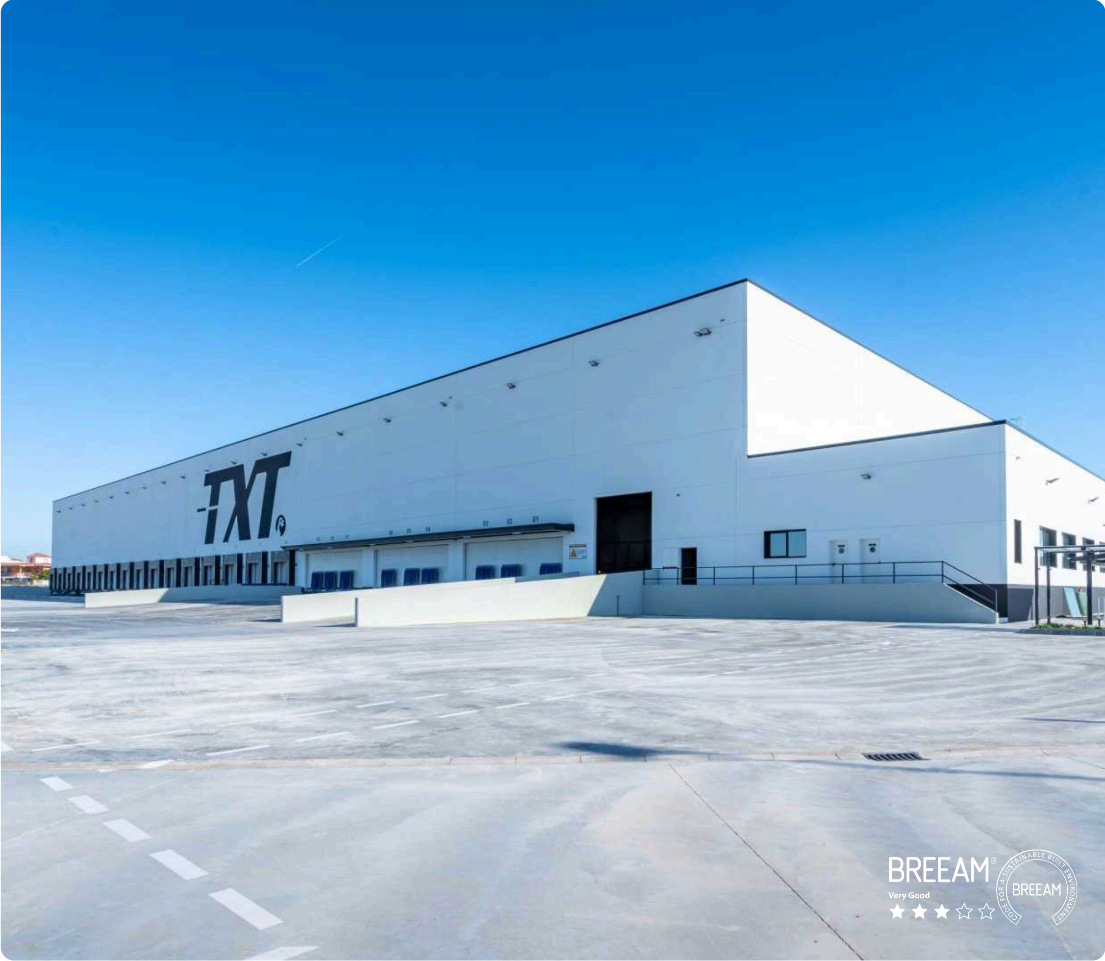
ACCOLADE FUNDS PARK SEVILLA
