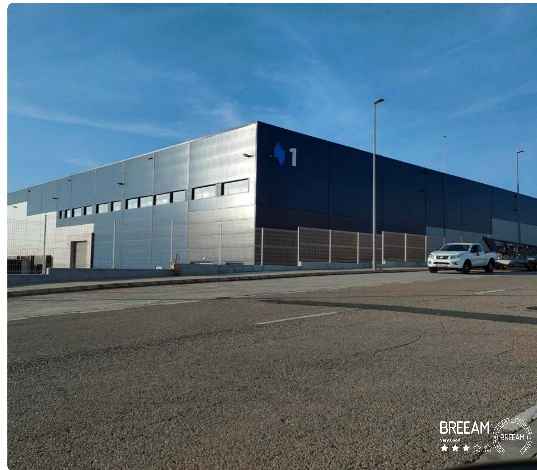
ACCOLADE FUNDS PARK VALENCIA PICASSENT
