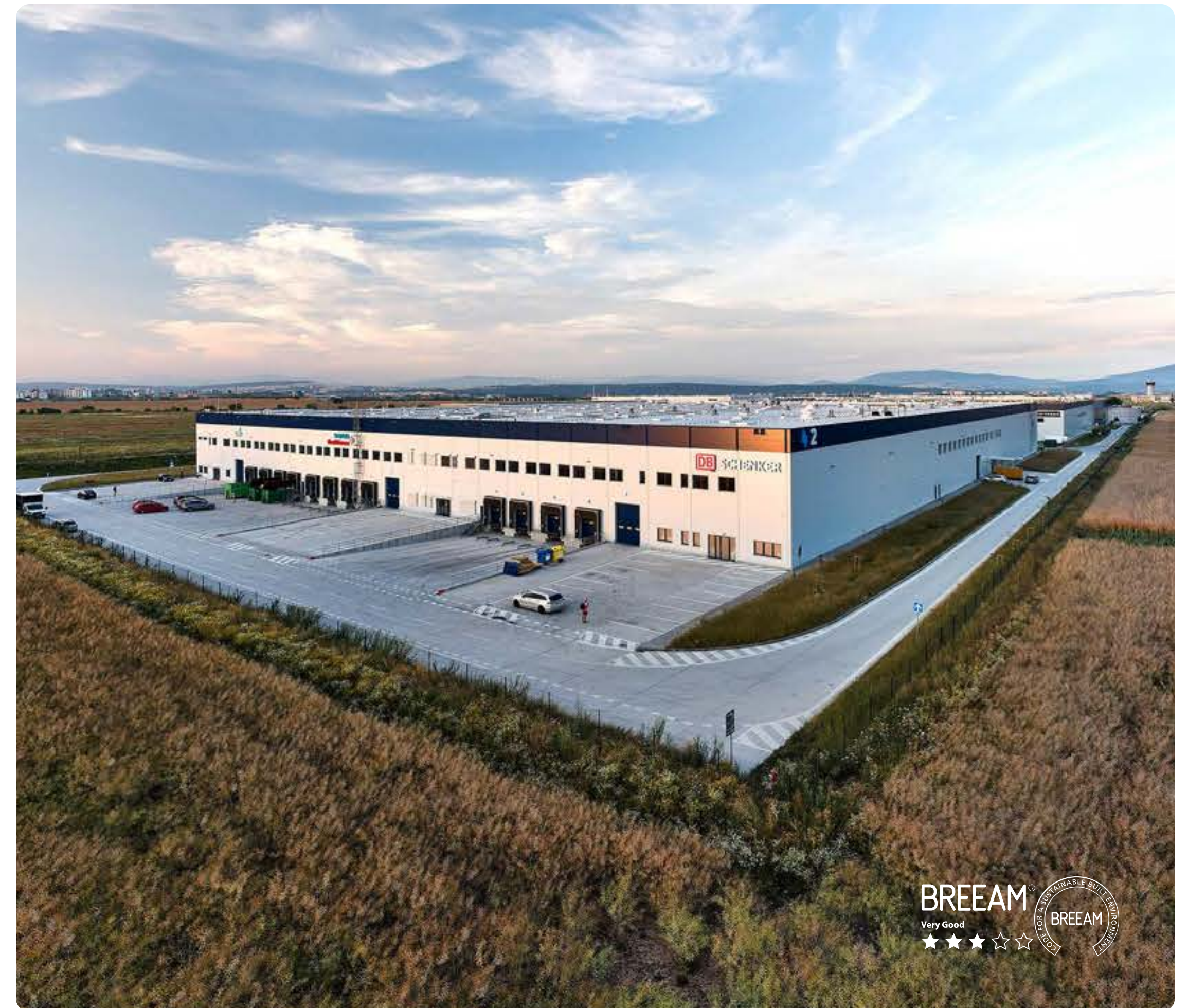
ACCOLADE FUNDS PARK KOŠICE AIRPORT
