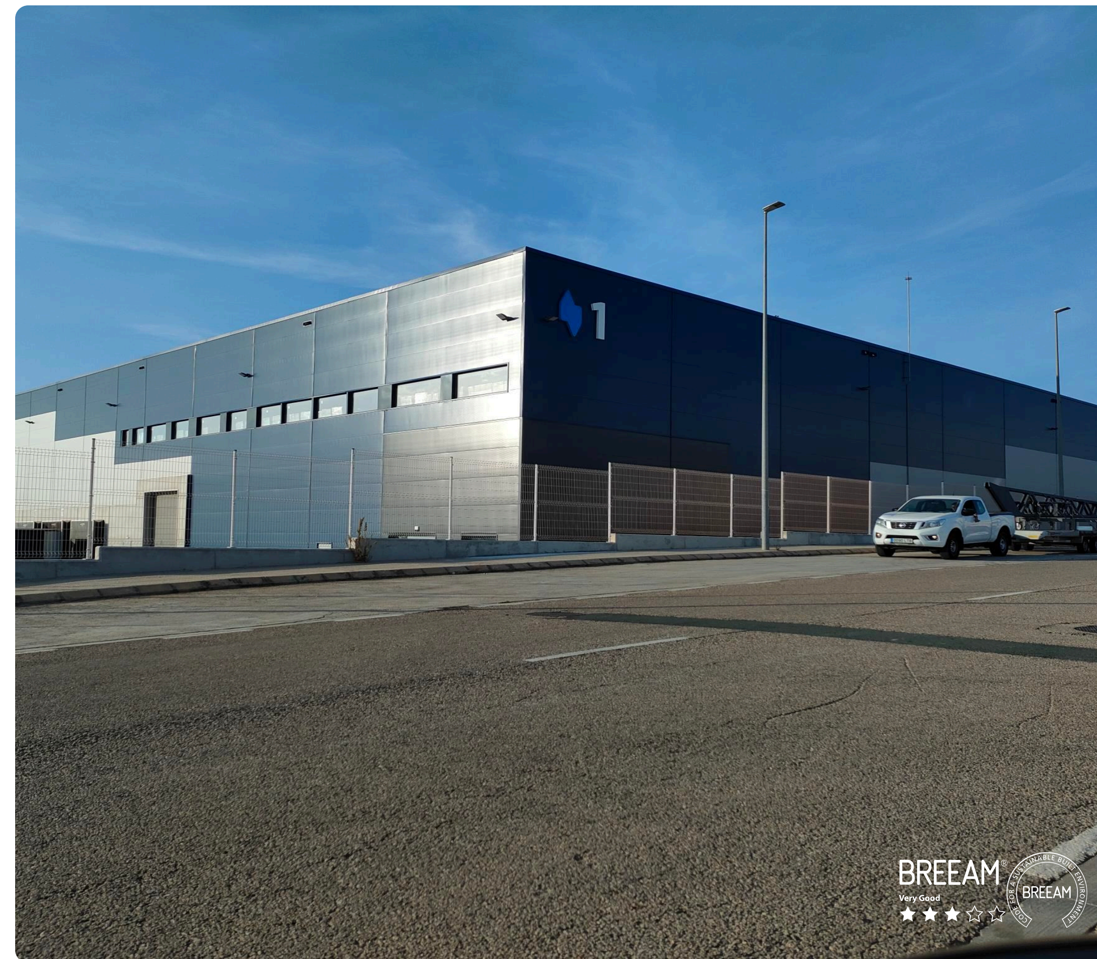
ACCOLADE FUNDS PARK VALENCIA PICASSENT
