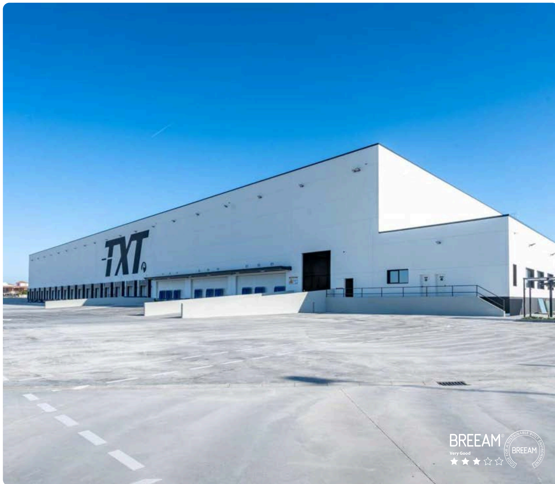
ACCOLADE FUNDS PARK SEVILLA
