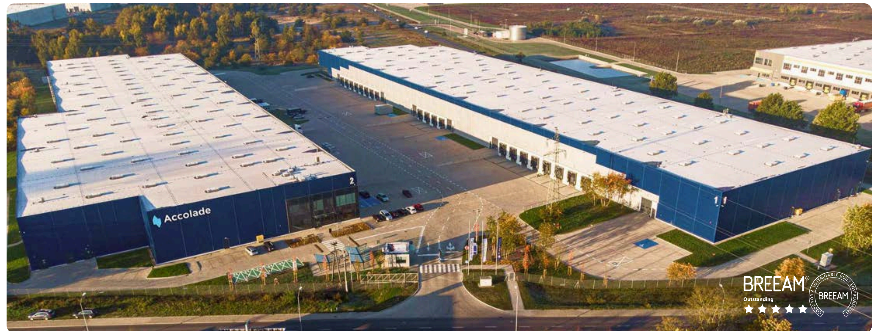
ACCOLADE FUNDS PARK SZCZECIN III
