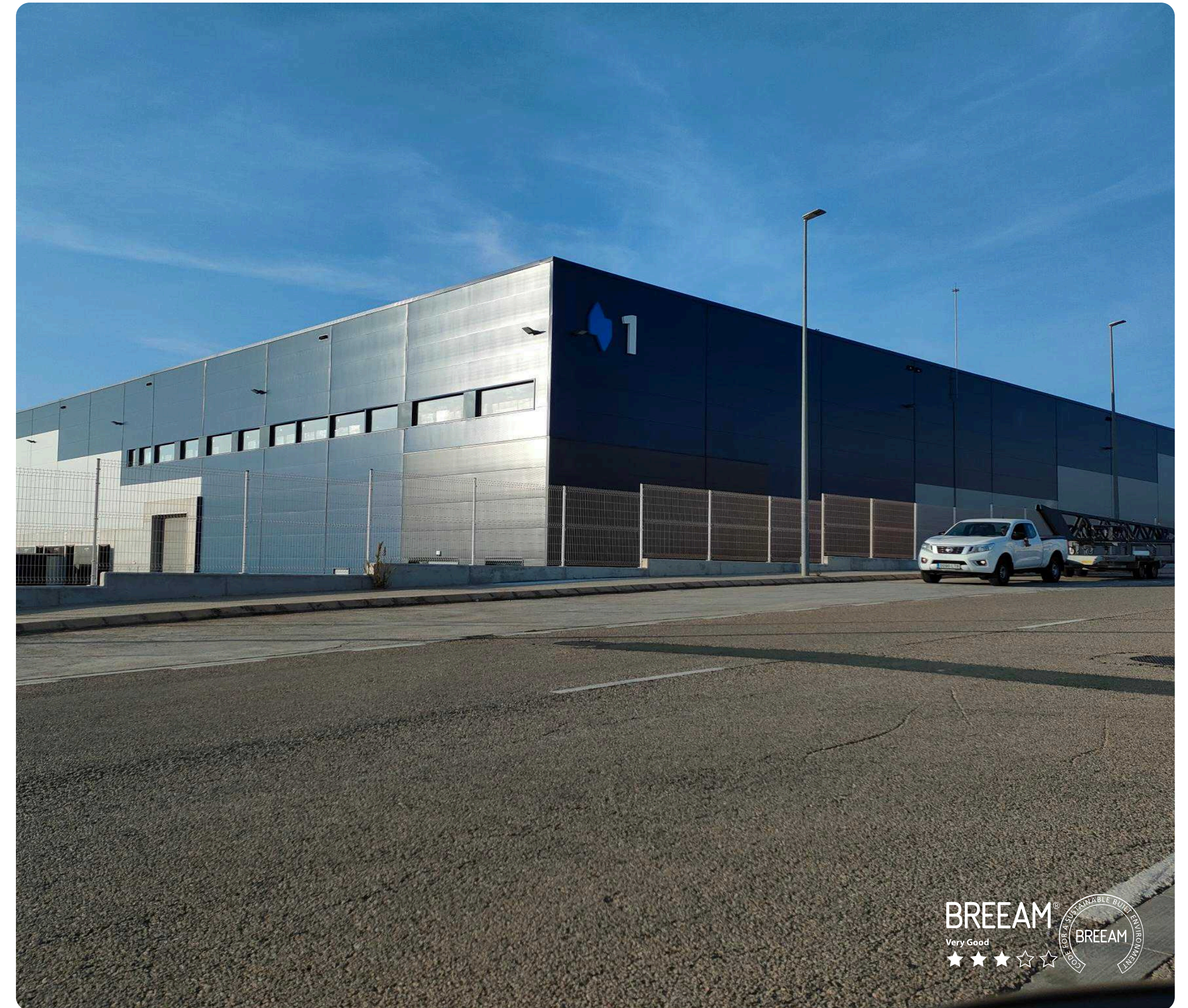
ACCOLADE FUNDS PARK VALENCIA PICASSENT
