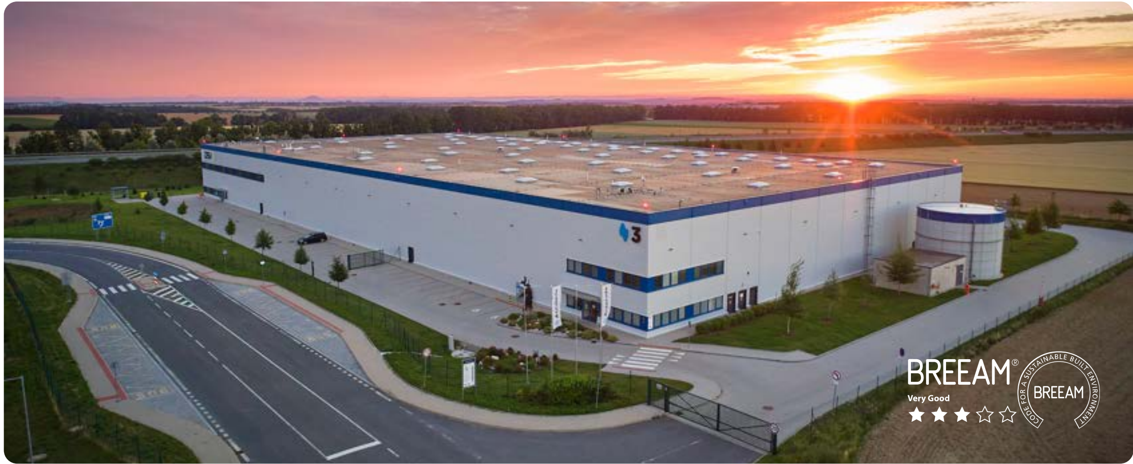
ACCOLADE FUNDS PARK PRAGUE AIRPORT II
