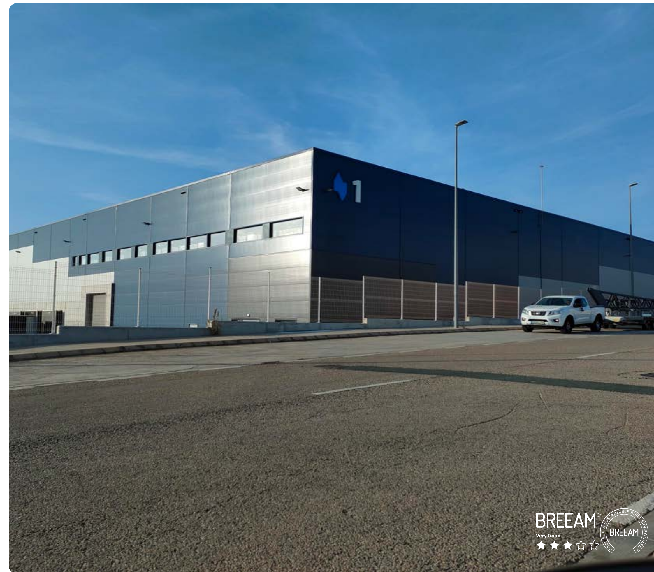
ACCOLADE FUNDS PARK VALENCIA PICASSENT
