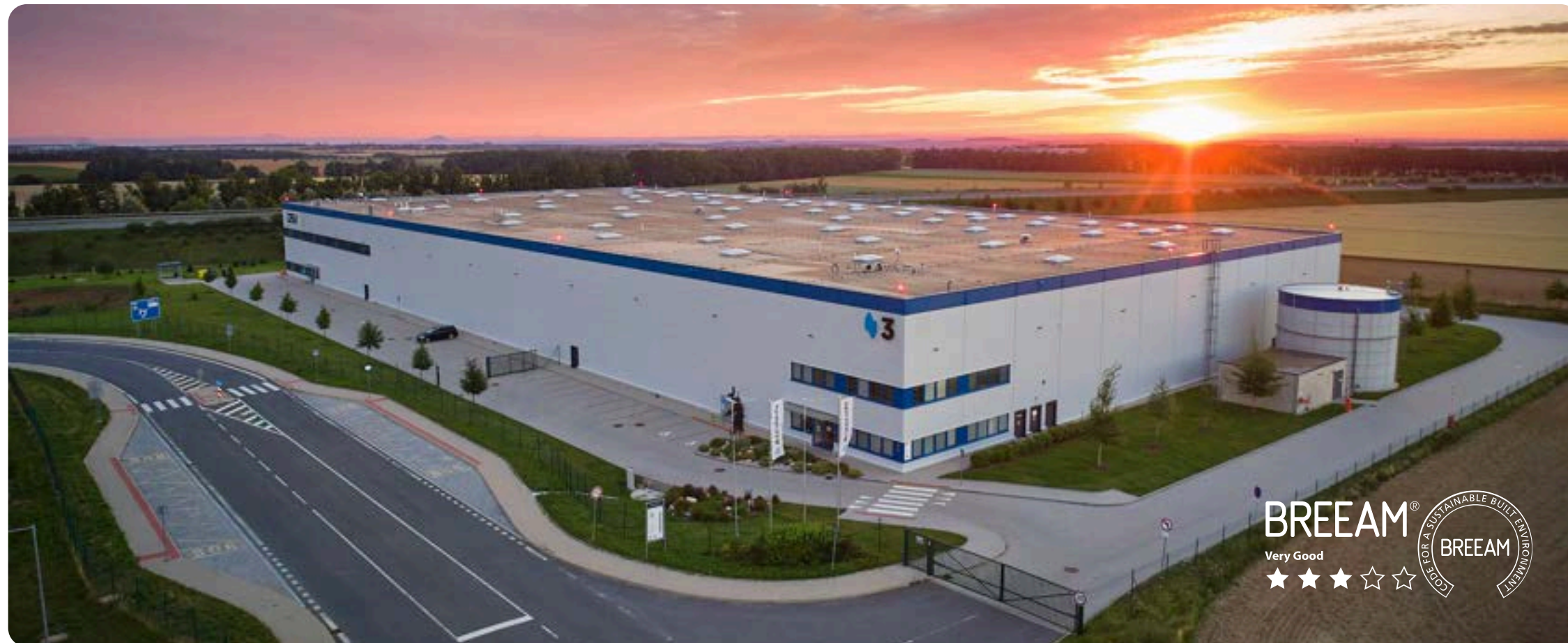
ACCOLADE FUNDS PARK PRAGUE AIRPORT II
