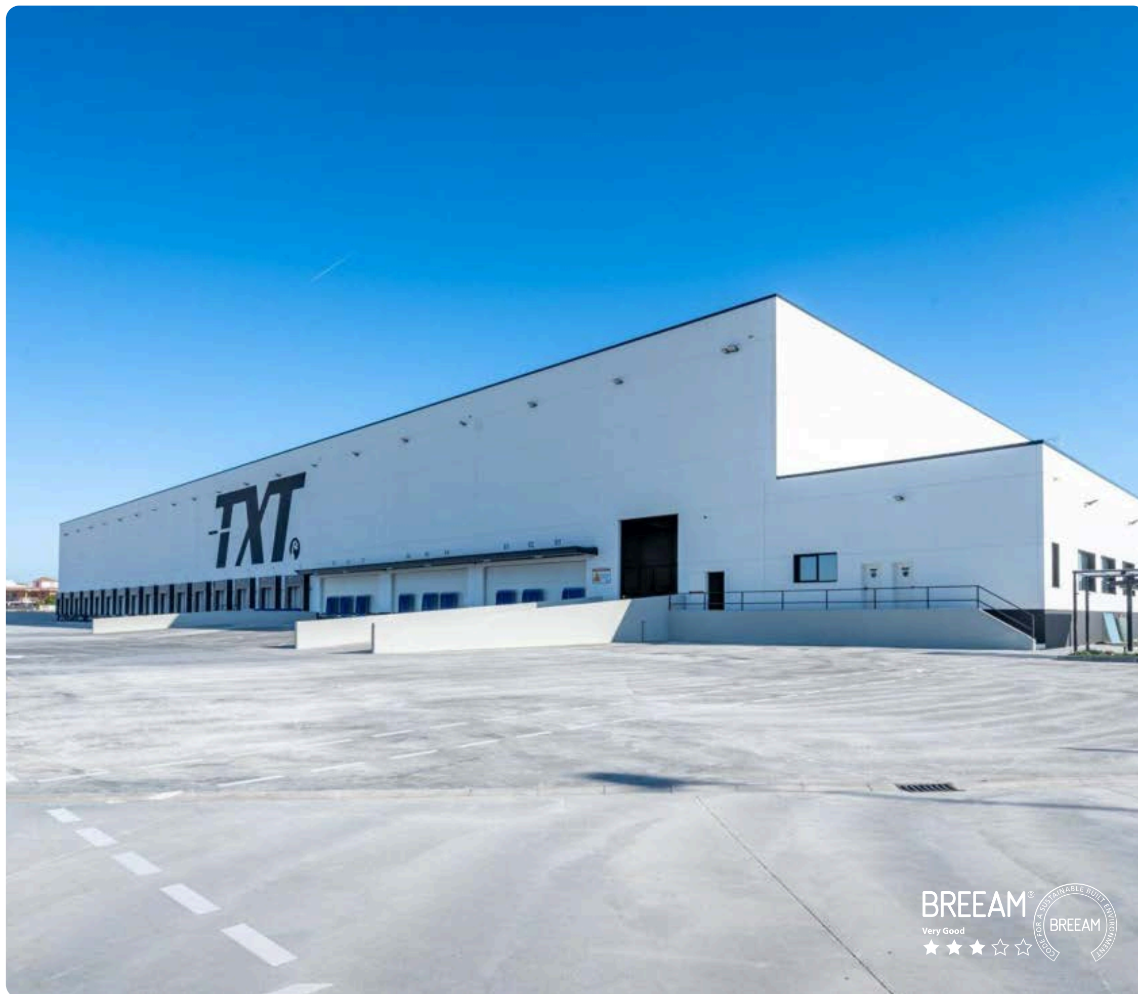
ACCOLADE FUNDS PARK SEVILLA
