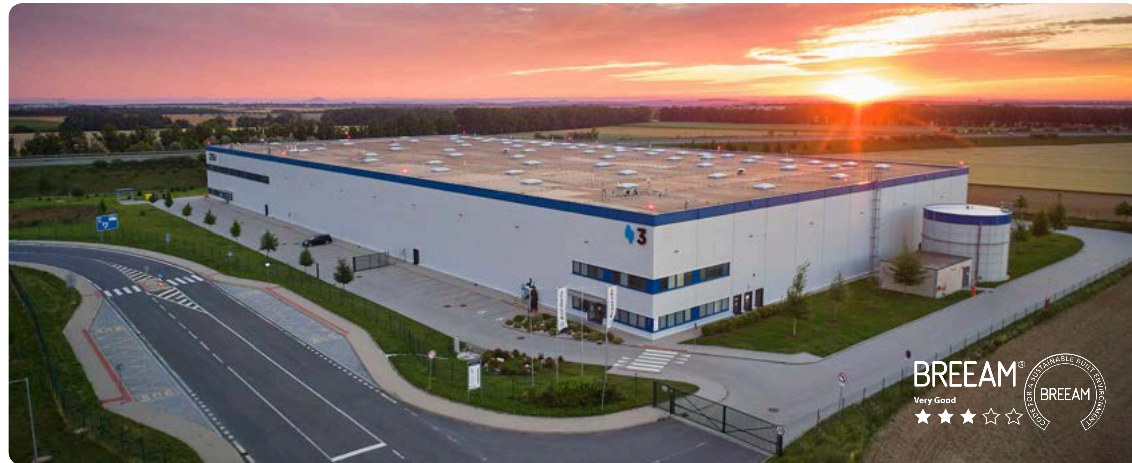
ACCOLADE FUNDS PARK PRAGUE AIRPORT II
