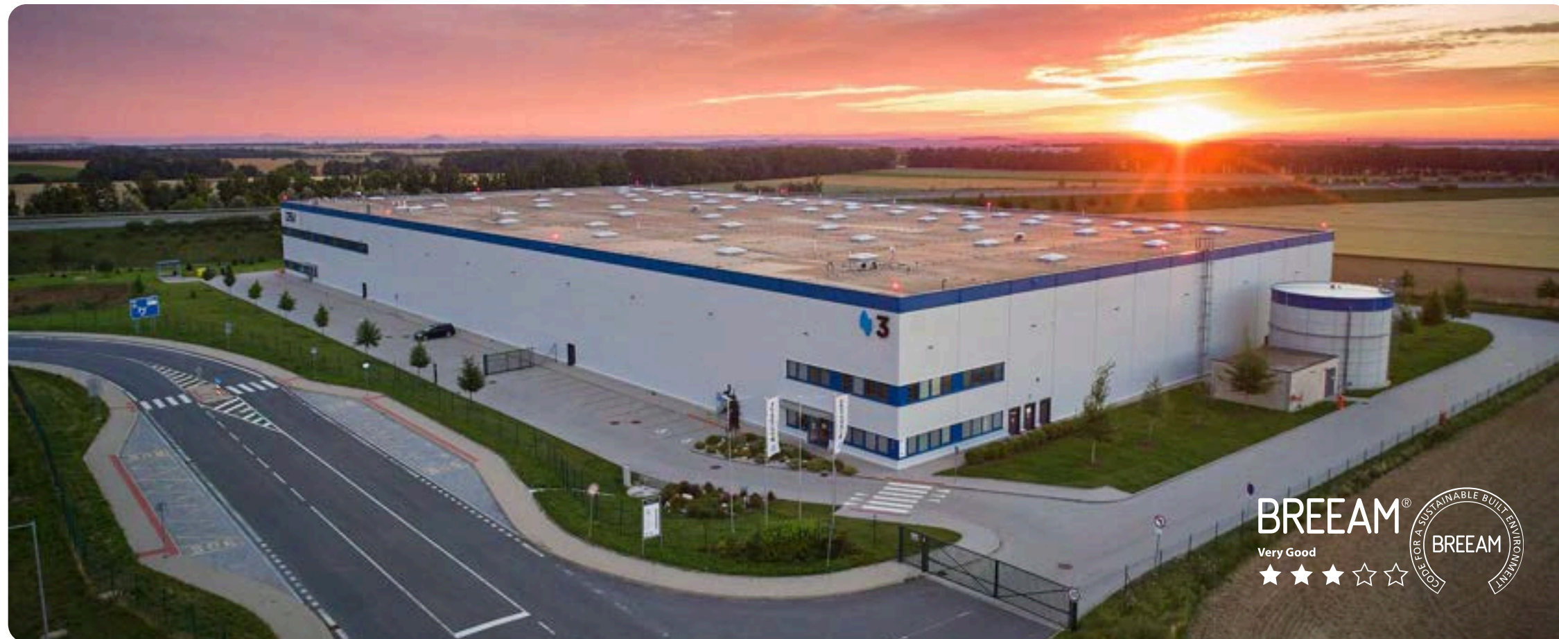
ACCOLADE FUNDS PARK PRAGUE AIRPORT II
