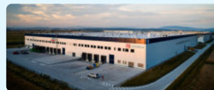
ACCOLADE FUNDS PARK KOŠICE AIRPORT
